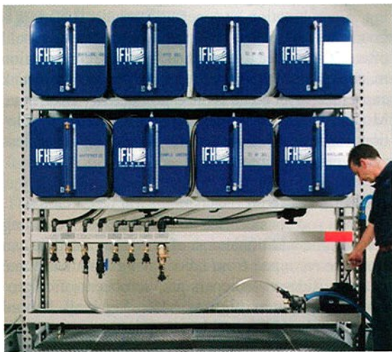
Fig. 2. An eight-container storage and dispensing system.
